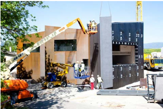
The new research and archive centre currently under construction in Penthaz
